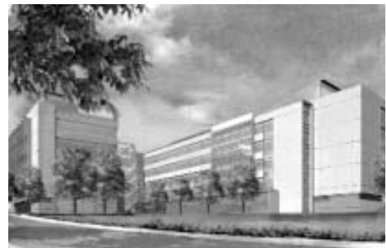
Health Sciences Building view from the northeast.
